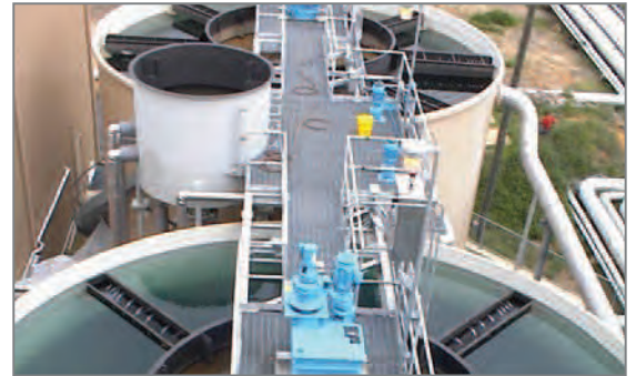
Industrial Surface Water Clarification
