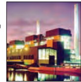
Eraring Power Station, NSW, Australia Reclaiming 2 MGD (peak flow) (7,500 m3/day)
